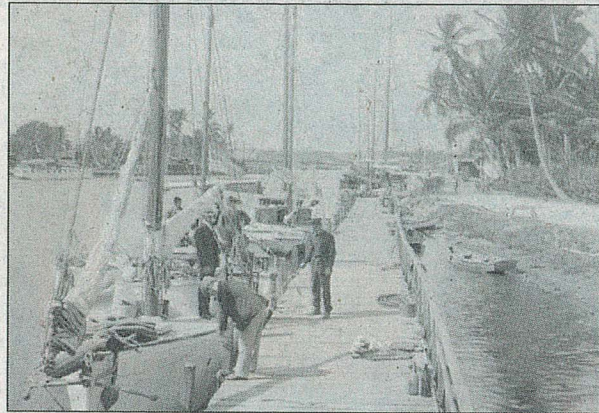
AT SITE OF PLANNED RIVER LANDING DEVELOPMENT, IN 1940S
