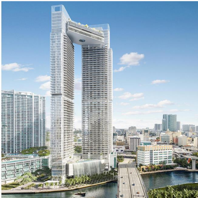
one river point features two symmetrical towers joined by a glass skybridge all images © KAR properties
