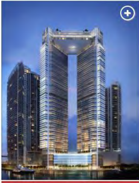
One River Point's towers will be joined by a three-story glass sky bridge at the top.
